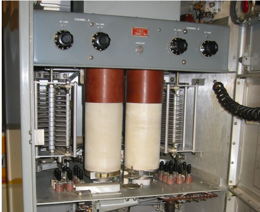
Figure 3. PA Compartment with Dual 4CX1500Bs and Cooling Chimneys in Place
